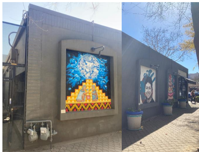
Tertiary (west) façade, composite view facing southeast. Source: ESA, 2024.
